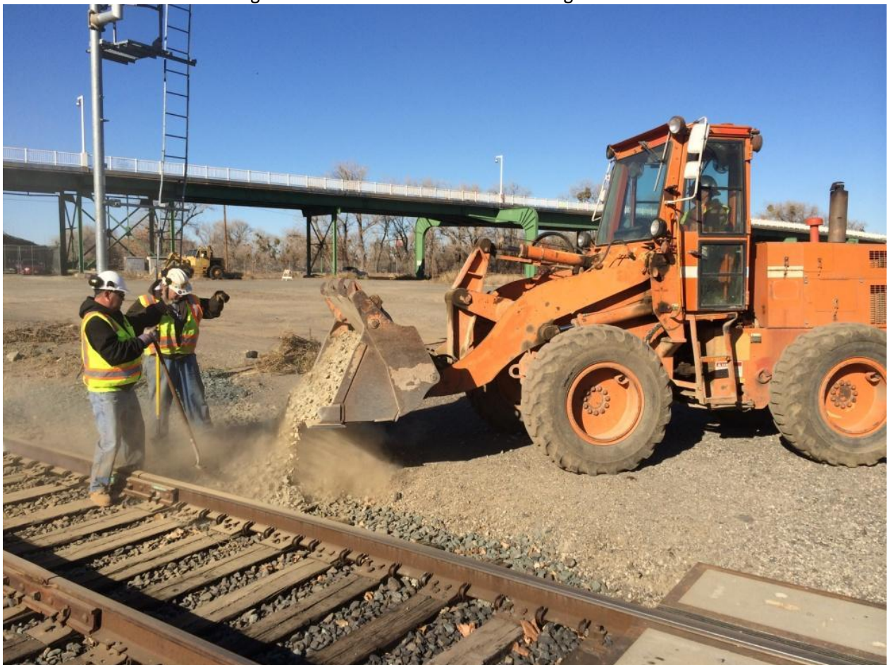
Taka and Mike F. show Mike H. in the loader where to fill-in the ditches near the signal mast
